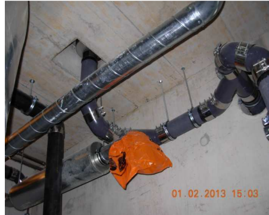
b) MLK - special cast iron drainage system, acid and greaseproof (manufacturer as above)
