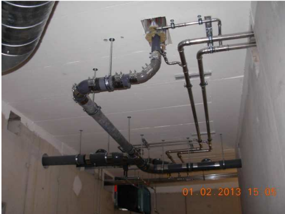
b) MLK - special cast iron drainage system, acid and greaseproof (manufacturer as above)
