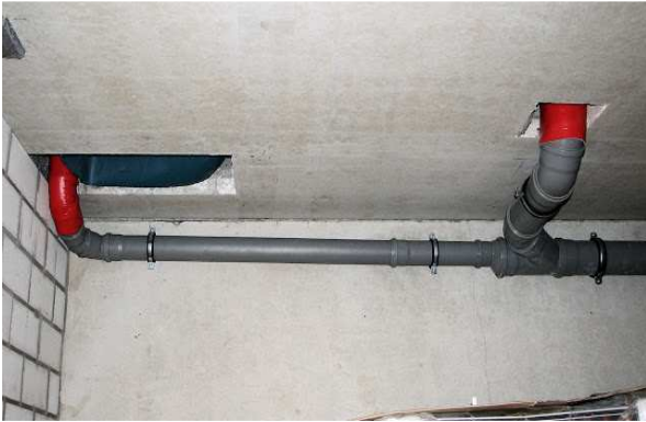
d) HT - plastic socket drainage system (various manufacturers)
