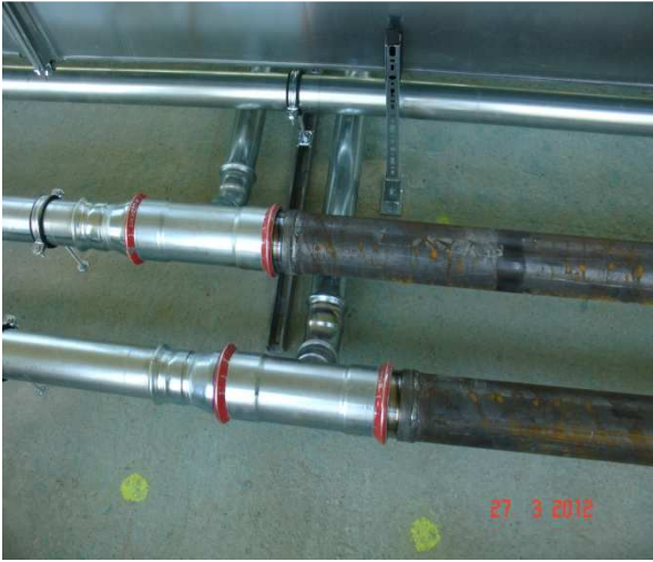
b) Installation of black steel pipes welded by gas or electrically (various manufacturers)
