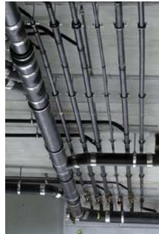
c) Silent BD20 - plastic drainage system, low-noise (manufacturer Geberit)
