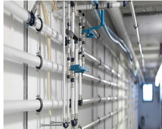
c) AL-Pex systems - aluminum-plastic composite crimped system (various manufactures)
