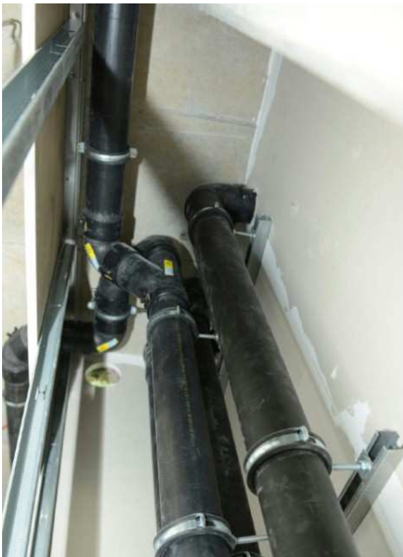
c) Silent BD20 - plastic drainage system, low-noise (manufacturer Geberit)
