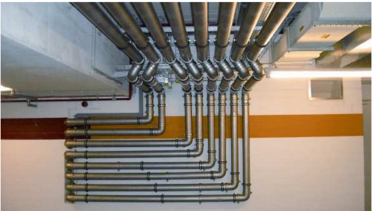
e) Stainless steel socket system (manufacturer e.g. Blücher)
