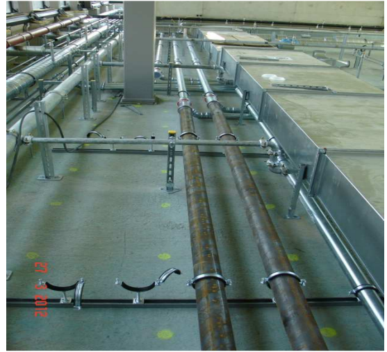
b) Installation of black steel pipes welded by gas or electrically (various manufacturers)
