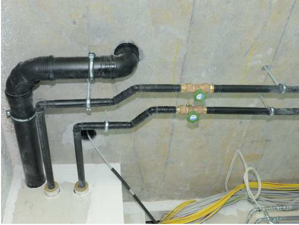
d) HT - plastic socket drainage system (various manufacturers)
