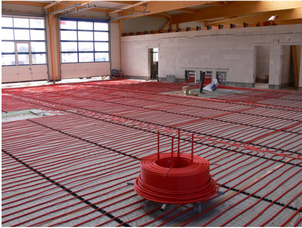
c) Under-floor heating pipes AL-Pex, Rehau or Mepla
