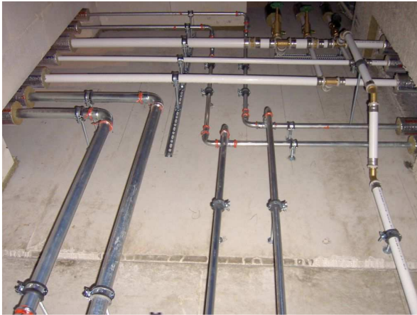
c) AL-Pex systems - aluminum-plastic composite crimped system (various manufactures)
